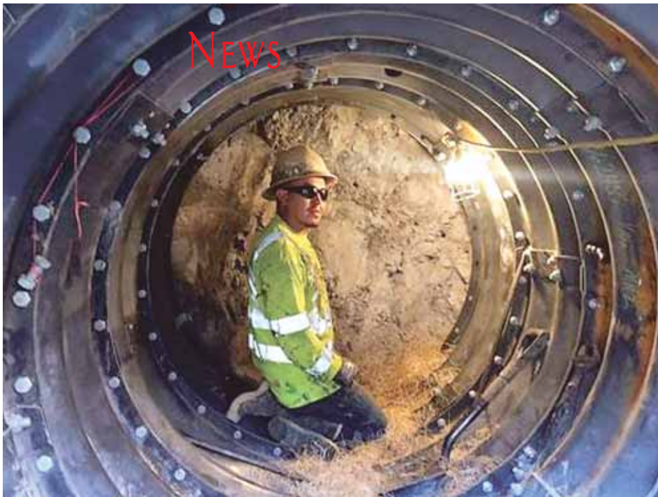
PHOTOS COURTESY OF CAPITAL RAIL CONSTRUCTORS A CRC worker kneels in the tunnel where he is hand mining to carry utilities to and from the Silver Line Phase 2.
