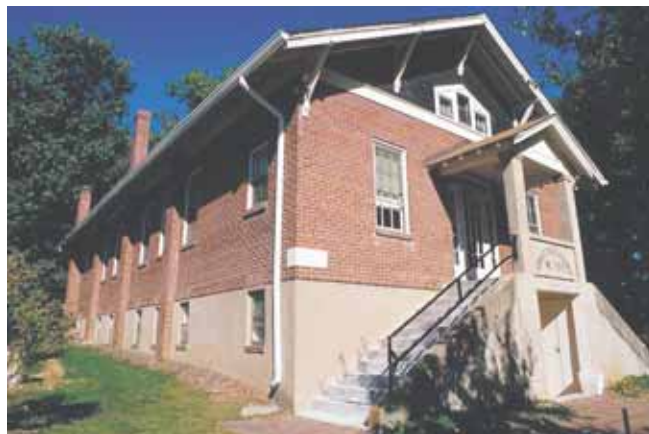
The Grange Hall was built in 1929. The Grange and its grounds were sold to the Park Authority in 1981.
