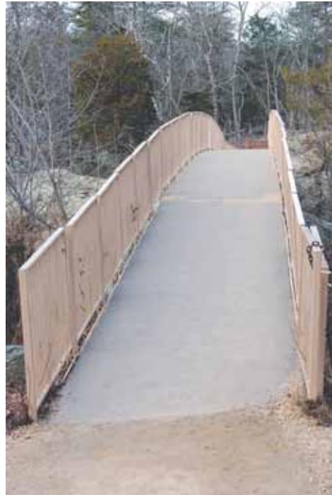
The railings are taken off when the river floods to reduce damage to the bridge. The connections to the railings will be replaced to make the railings safer and easier for the rangers to remove during flooding.
