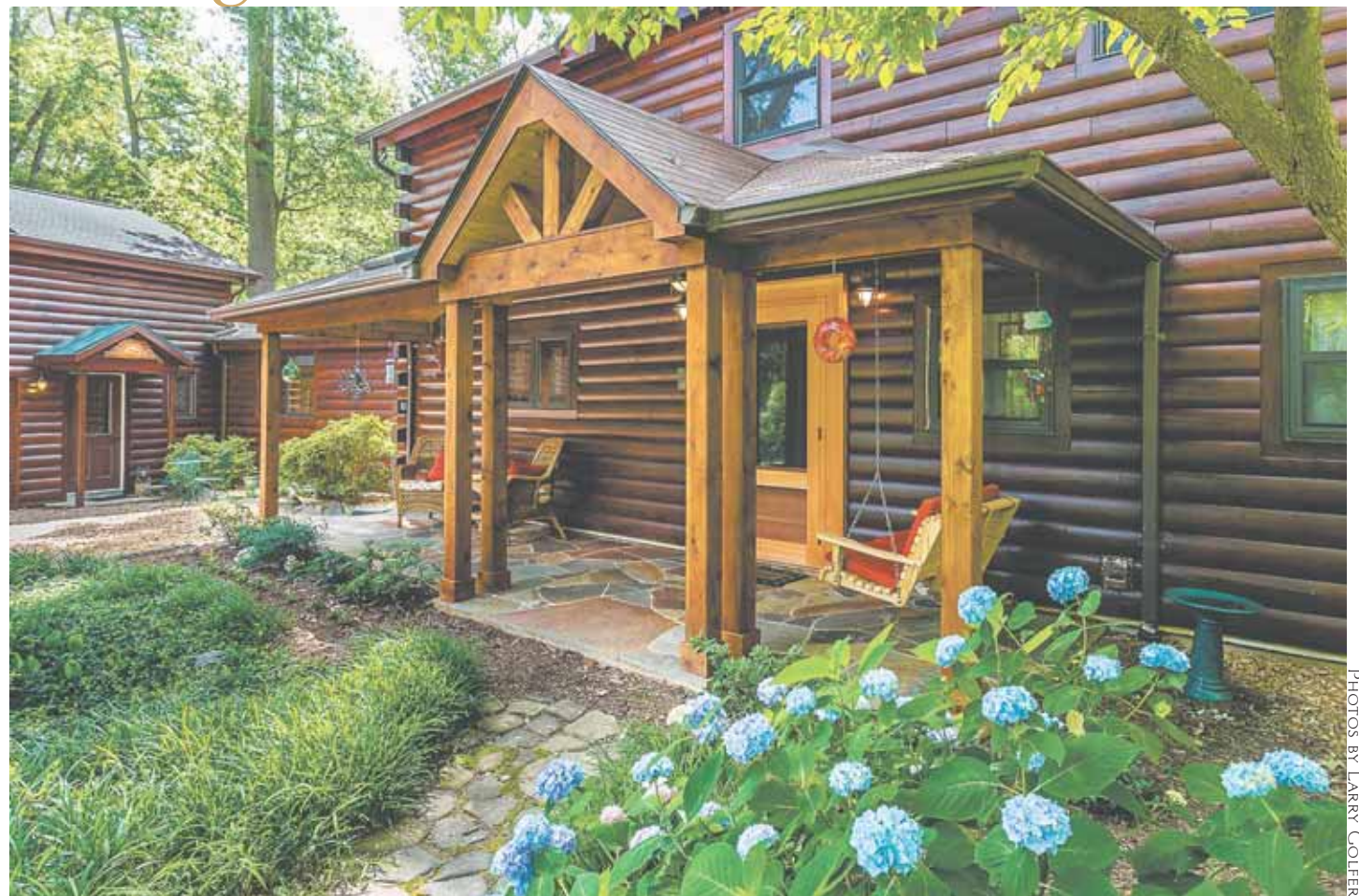
Rough-hewn timbers — the handiwork of Foster master carpenter Mike Borman — is integral to the aesthetics of a new front elevation that is both inviting and whimsical. Red cedar trim and molding provides sympathetic color accents.
