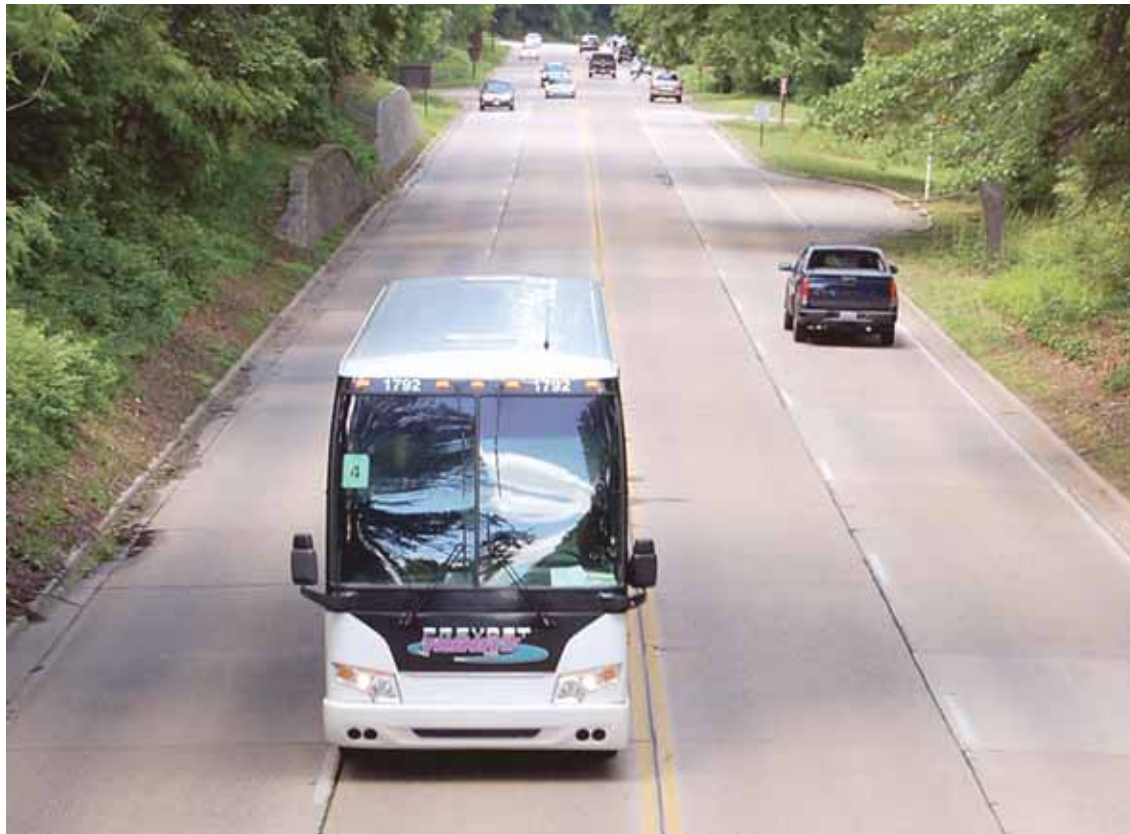
The Parkway's center lanes measure only nine feet wide, or 108 inches. The tour bus pictured is 102 inches wide. The outer lanes are 11 feet wide. Neither lane dimension meets current Virginia highway standards.
