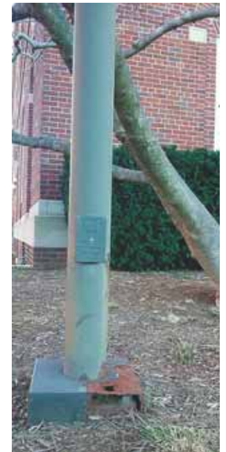
Photo of lamp pole located on federal property in the 200 block of South Washington and Prince Street.
