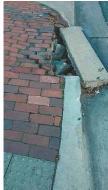
Photo of damaged sidewalk/curb at the intersection of 400 and 600 block of South Washington and Wilkes Street.
