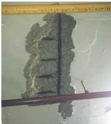
**Concrete deterioration exemplifies numerous problems, not least structural, with City Hall's underground parking garage. Expansive drainage, waterproofing and other repairs will cost an estimated \$6.5 million over FY19-27.**
