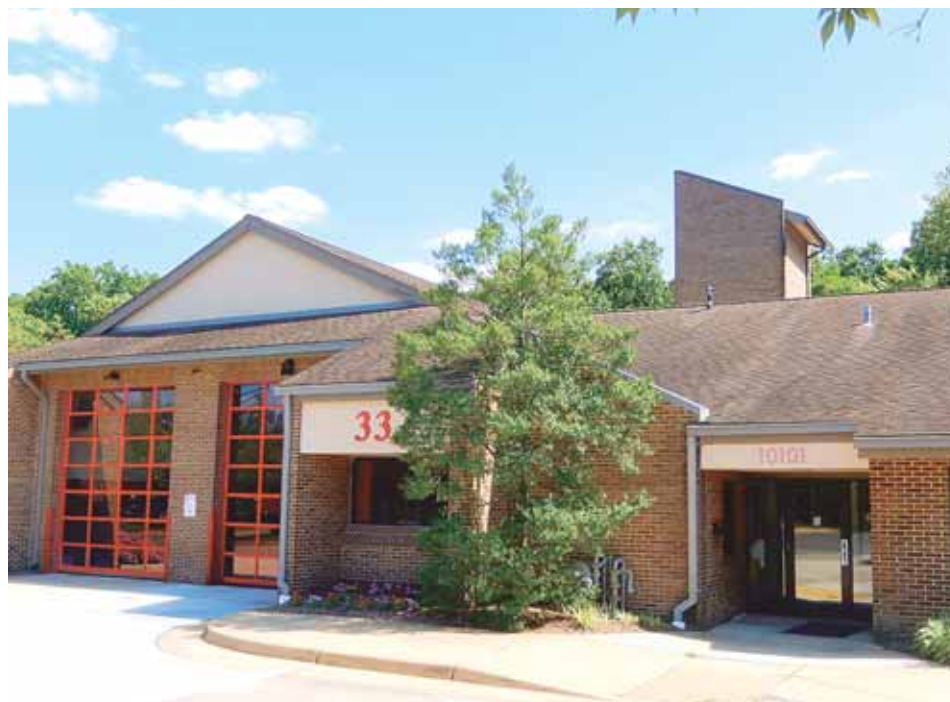
Fairfax Fire Station 33 is going to be demolished and rebuilt.
