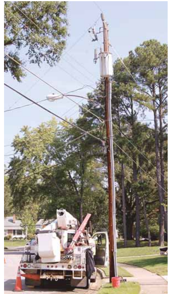
The single power line atop the pole, the transformer and the triple power lines will be removed in September. Phone and cable lines are below the power lines. The streetlight will be powered from below.
