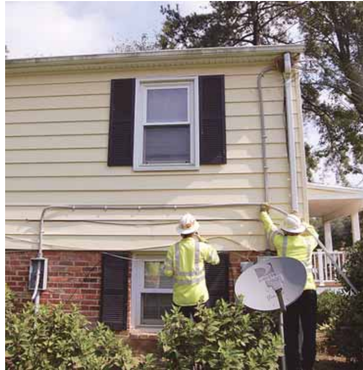
Two men from Dominion contractor Will-Bros, Allister Pollard, left, and Mike Creed, connect a Conover Place residence to a new underground power distribution line at far left.
