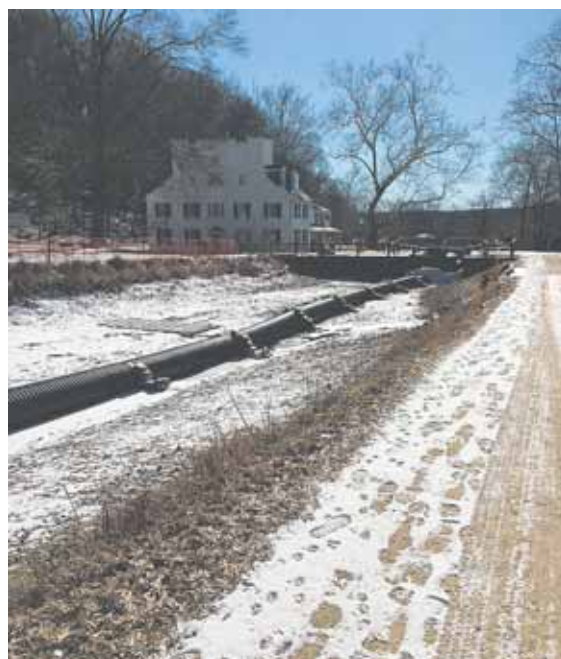
A pipe on the bed of the C&O Canal by Great Falls Tavern keeps water from filling the canal during construction.
