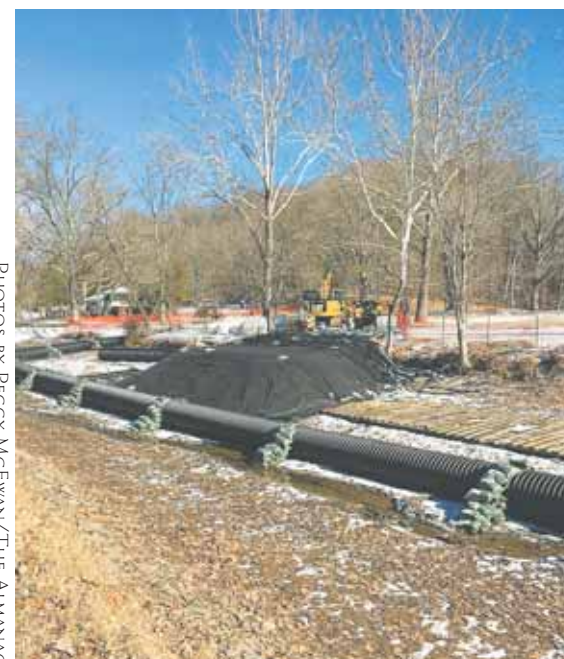
Workers construct a temporary causeway across the C&O Canal near Great Falls Tavern.
