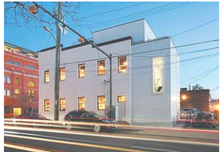
The 130 N. Fayette renovation project.
