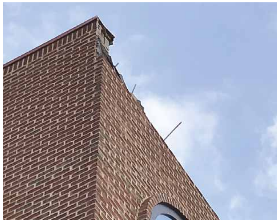
The area on the right-hand side of the three-story commercial building at 754 Elden Street in Herndon shows where the concrete decorative cornices rested up until Saturday, June 9 when they fell for unknown reasons.
