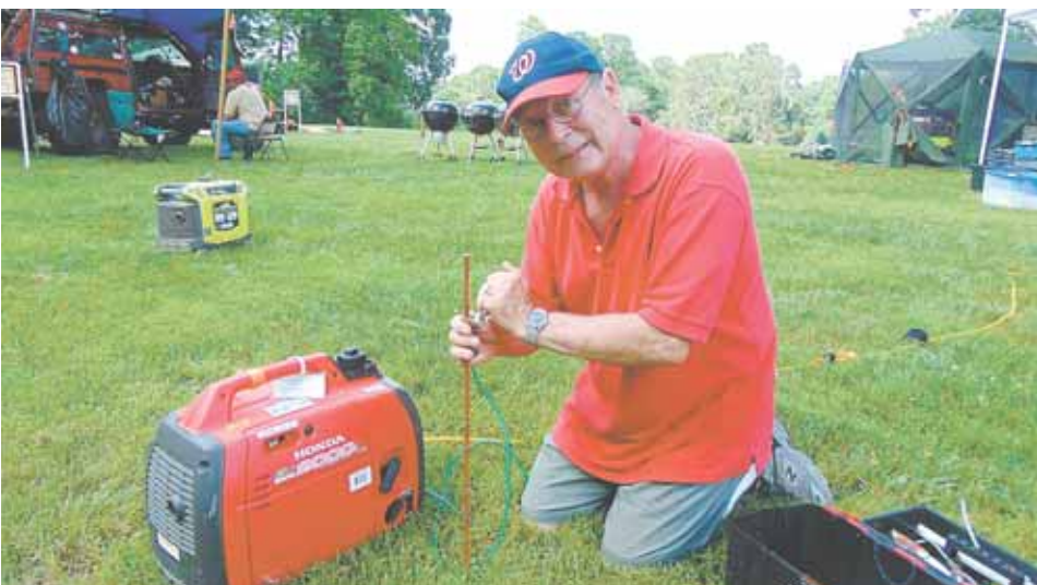
Mike Aimone of Fairfax installs a ground conductor on a portable generator.
