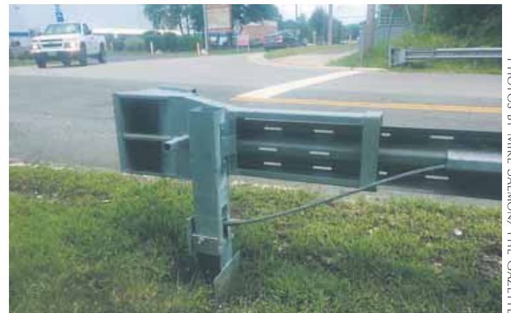
This is what the guardrails look like before being hit, with the built-in shock-absorbing features in plain sight.
