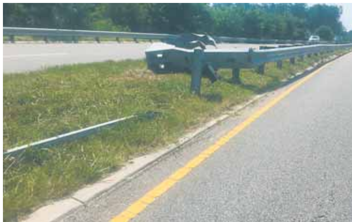
Along Jeff Todd Way in Mount Vernon, a guardrail in the center island was hit but buckled the way it was intended.
