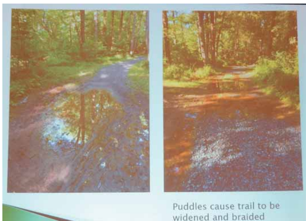
These photos show degradation of the gravel trail after a rain.
