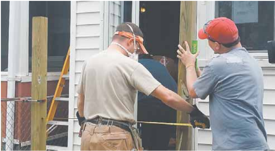
Rebuilding Together's volunteers at work.
