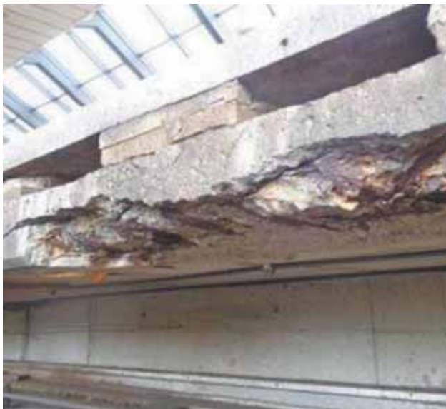
Structural damage at King Street Metro Station.
