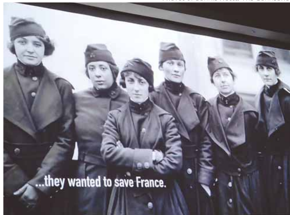
Women in the U.S. Army Signal Corps served in France as switchboard operators during WWI.
