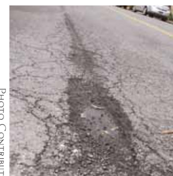
Asphalt seams are a good place for the freeze and thaw process to start, like this one at Duke and Pitt streets.
