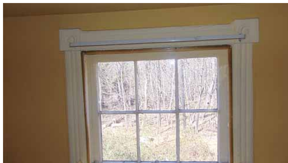
The Hannah P. Clark house features windows with bullseye moldings.
