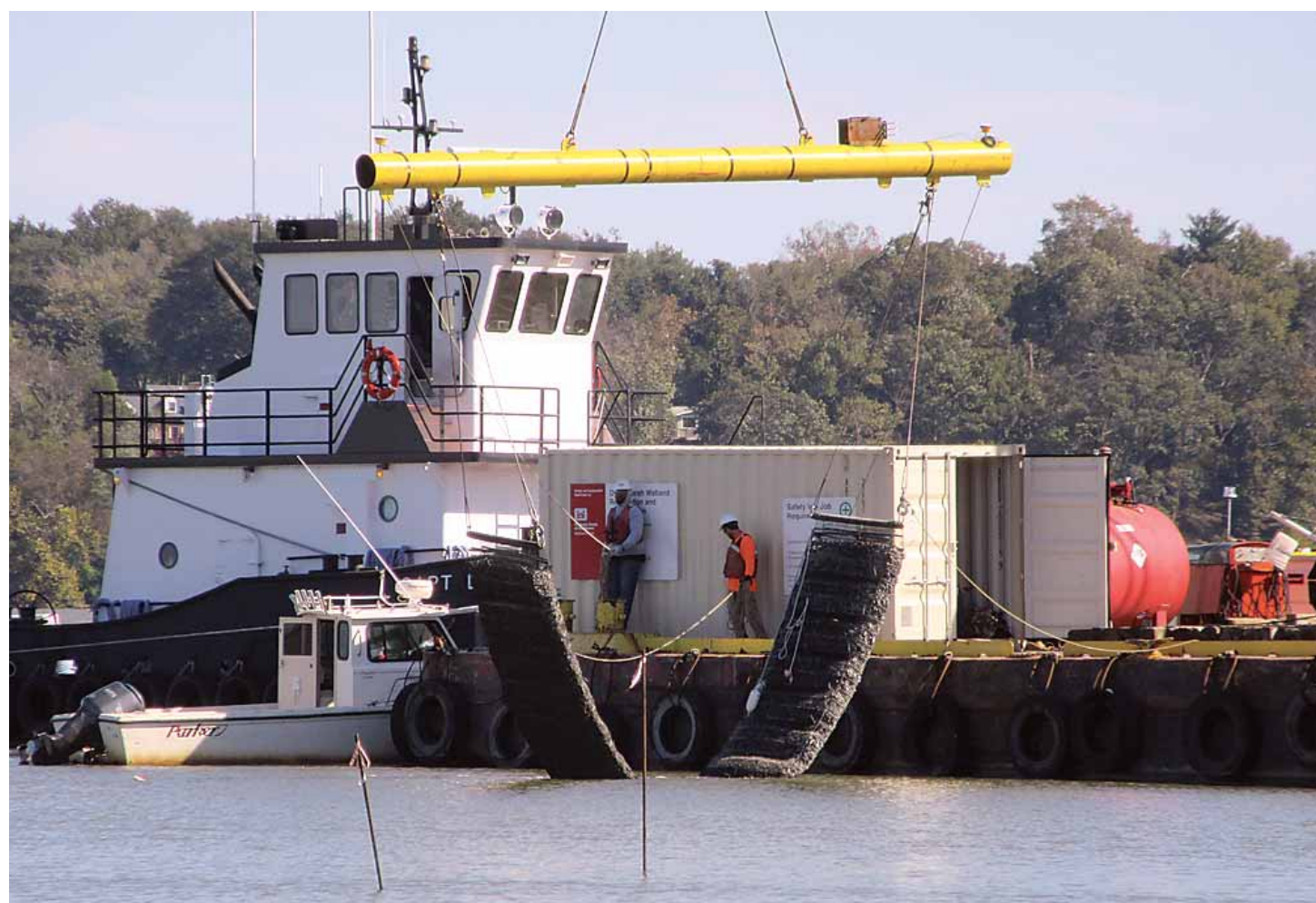
SEE RISING WATERS, PAGE 3 Cranes lower marine material to the river bottom to form the foundation of the breakwater.
