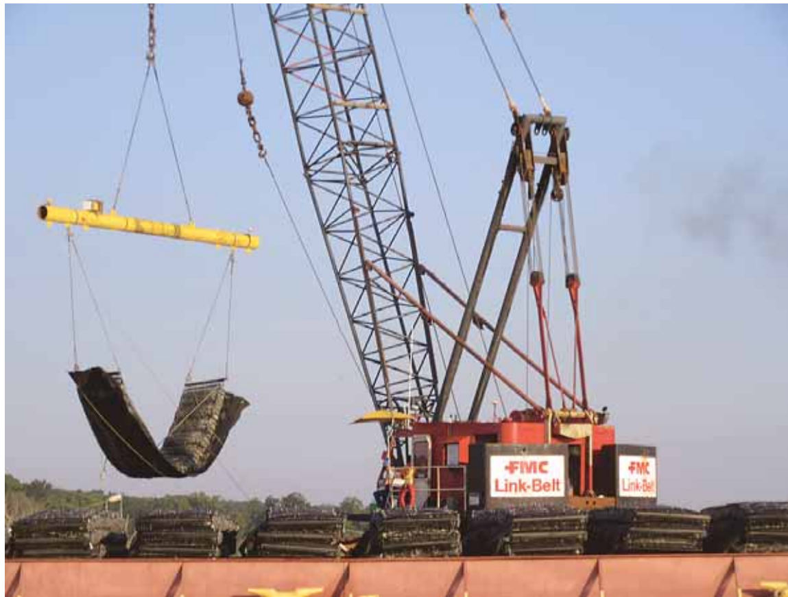
A crane lowers a marine mattress into the river to support the breakwater.
