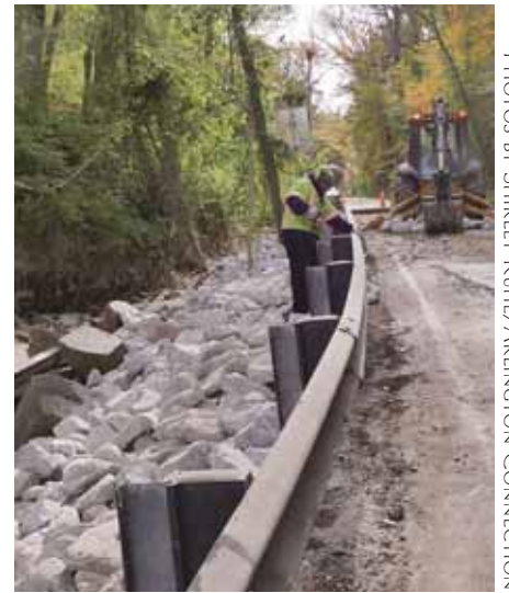
Bulldozers work to restore Chain Bridge Road which was blown up by a burst water pipe early Friday morning. The pipe burst just under where the bulldozer is working on Saturday morning, blowing the road apart, gushing down the side of the road and taking down the railing.
