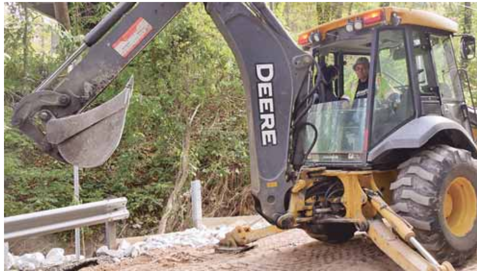
Bulldozers work to restore Chain Bridge Road which was blown up by a burst water pipe early Friday morning. The pipe burst just under where the bulldozer is working on Saturday morning, blowing the road apart, gushing down the side of the road and taking down the railing.
