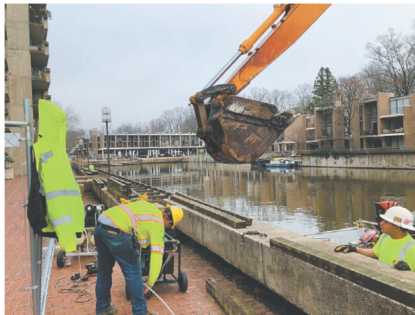
Steam shovel removing sediment sucked from underneath the Lake Anne Dock by hydraulic dredging equipment.
