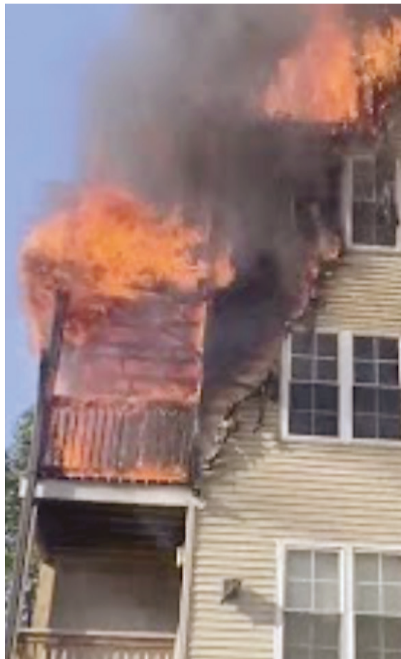
This fire at a Centreville apartment building was caused by fireplace ashes improperly discarded on a balcony.
