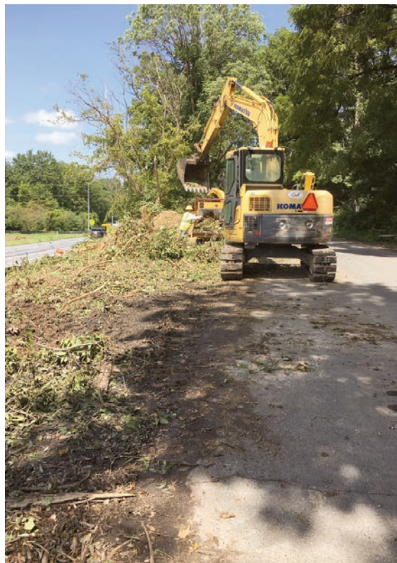
Trees and vegetation are removed along Braeburn Parkway above west bound lanes of River Road to make room for a reconstructed pedestrian path across River Road at Pyle Road heading time Whitman High School.
