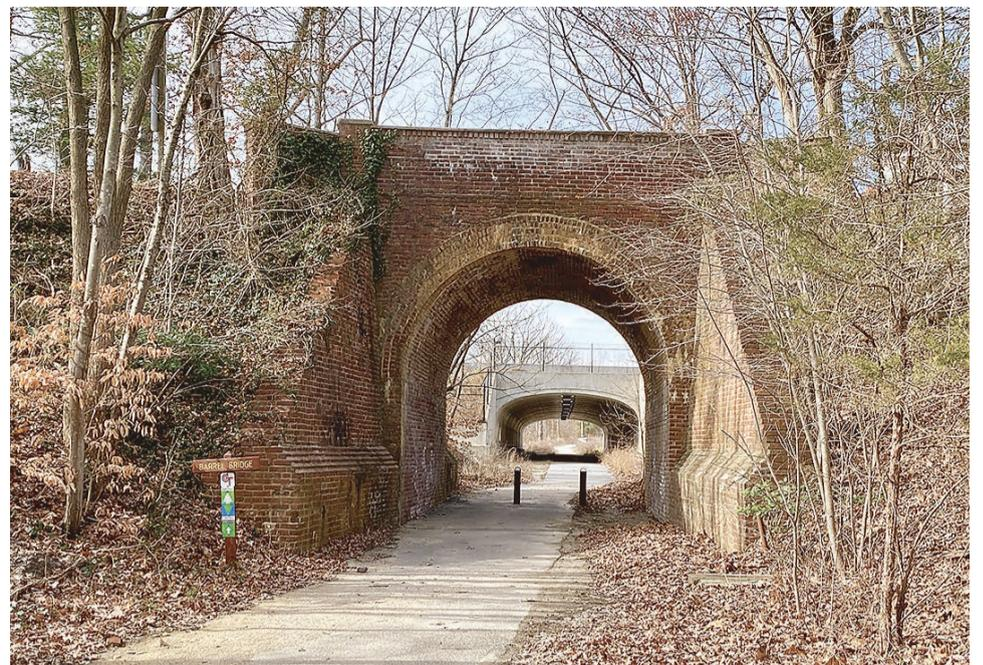
Barrel Bridge (Laurel Hill Park 8780 Lorton Rd, Lorton). Historic brick and masonry arched bridge built in 1946, outlines a new bridge (background) which replaced it for vehicular traffic.
