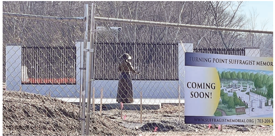
Site of the Turning Point Suffragist Memorial under construction with expected completion in Spring 2021.
