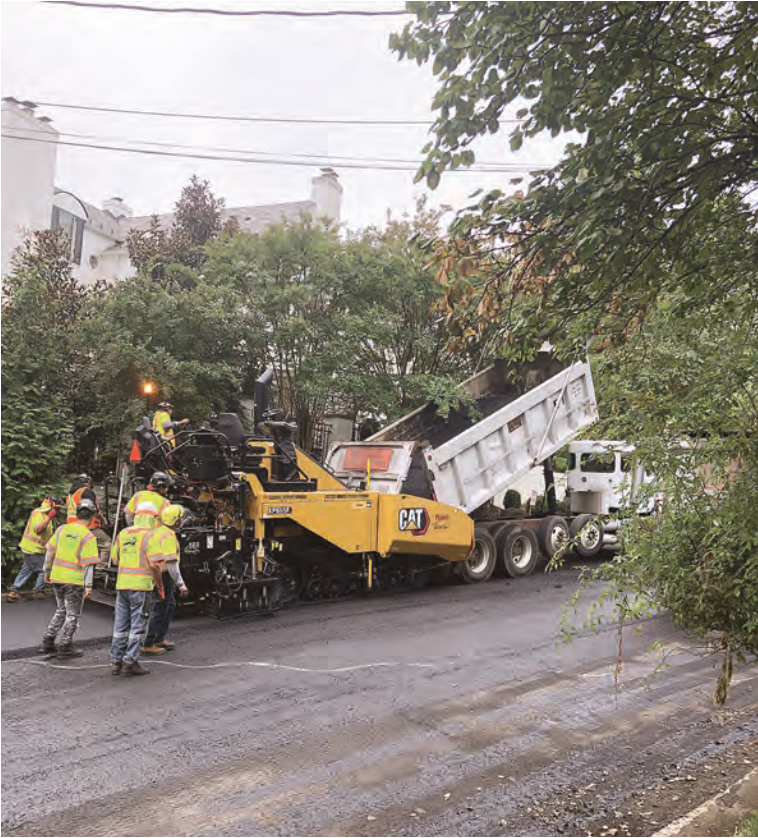
Truckload of hot asphalt goes down on the street.
