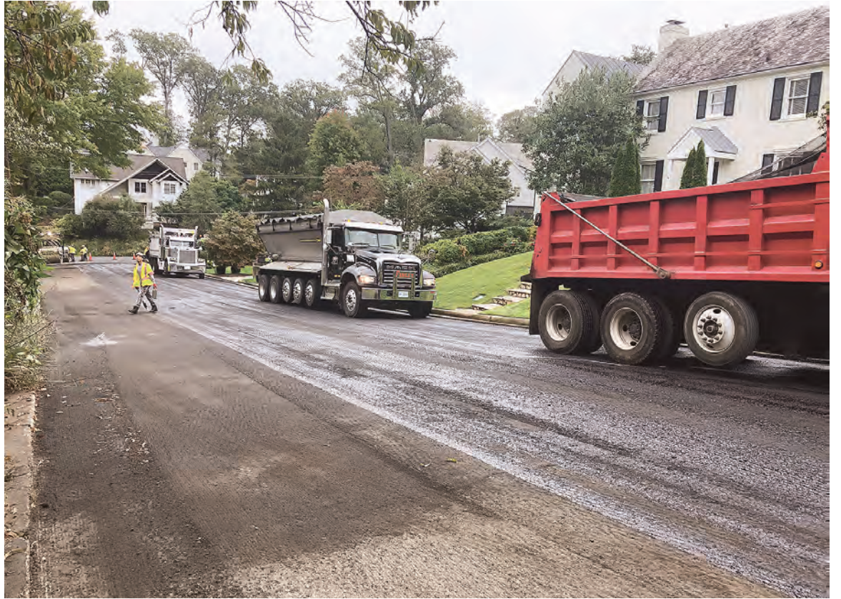
The scraped road gets ready for asphalt.
