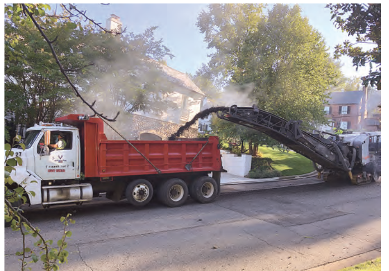
An Arlington street is scraped down as old asphalt is conveyed to trucks and sent for turning into RAP.
