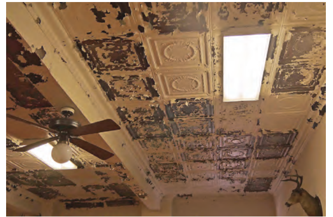
The ceiling in the Lodge Room has had repairs for numerous leaks but the historic tin squares on the ceiling are awaiting the appropriate and difficult historical renovation.
