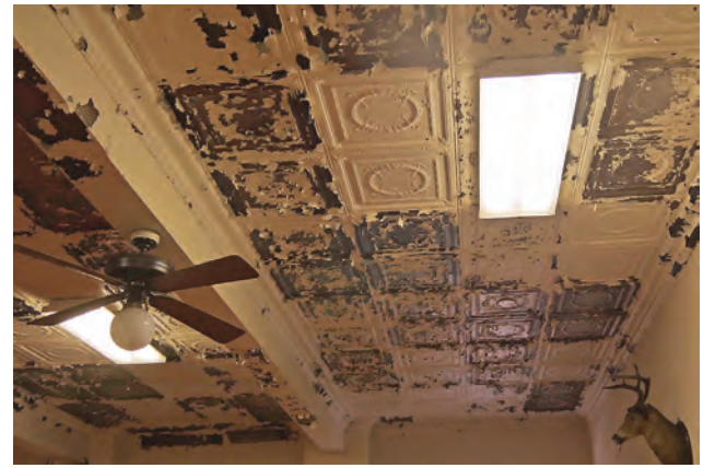
The ceiling in the Lodge Room has had repairs for numerous leaks but the historic tin squares on the ceiling are awaiting the appropriate and difficult historical renovation.
