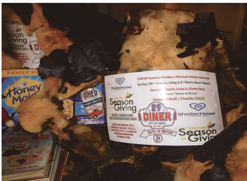
Juxtaposition: A poster for 29 Diner's "Season of Giving" is surrounded by blackened plaster and burnt insulation.
