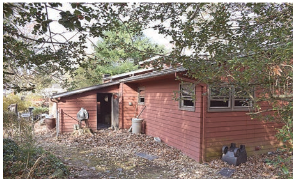
Damages as a result of this fire were approximately $37,500, Fairfax County Fire reported.
