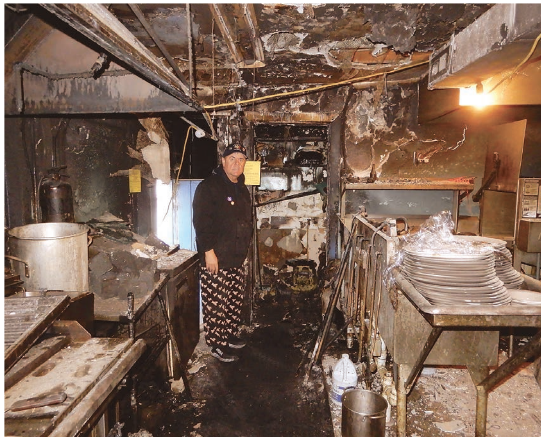
Owner John K. Wood inside the diner's destroyed kitchen. The fire started in the supply closet next to and behind him.
