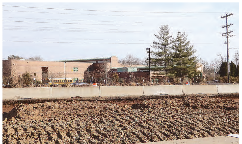
The widening project goes right by Centreville Elementary.
