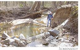
February 2008 at Snakeden Branch in Reston: Northern Virginia Stream Restoration Bank comprises approximately 11 miles of streams, poised to be restored using a phased approach. By project end, restoration of the stream utilized so called "natural channel design," raising the bed to reconnect storm flows with the floodplain.
