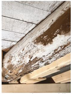
Basement restoration exposes peeled log construction used to minimize construction costs
