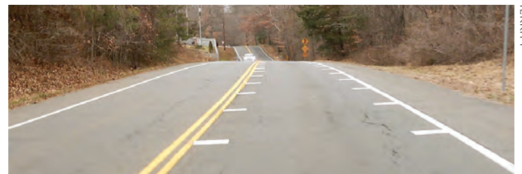
On the approach to the hill, these optical speed bars were installed recently to create awareness.
