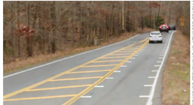
On the approach to the hill, these optical speed bars were installed recently to create awareness.
