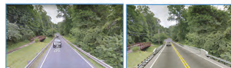
Springvale Road bridge (State Rt. 674) 2020 plan by VDOT: Before (single lane) and proposed two-lane, no median option.
