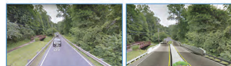
Springvale Road bridge (State Rt. 674) 2020 plan by VDOT: Before (single lane) and the proposed median option.
