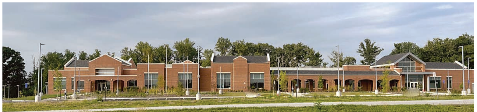
The new Lorton District Police Station and Animal Shelter near completion is expected to open in the Fall.
