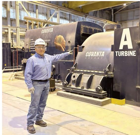
Covanta manager Don Cammarata, points out one of the plant's two turbine generators which convert steam to electricity.
