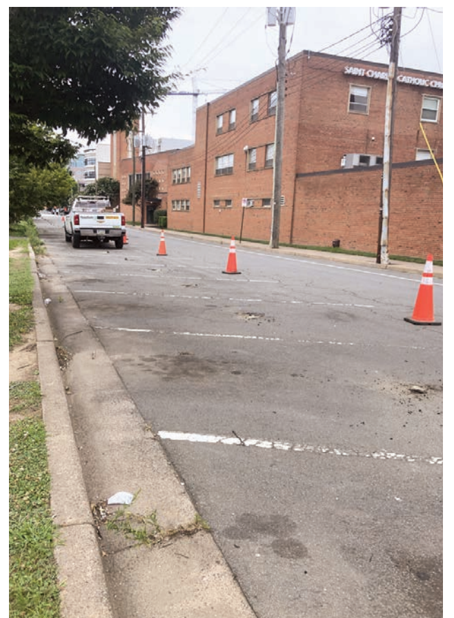
Contractor punching holes in the parking spots near Northside Social.
