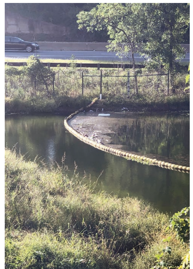
A barrier at the north end of the wetland keeps trash from continuing down the flow of Lubber Run.
