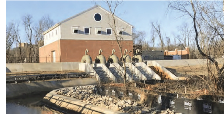
The Huntington Levee and Pumping Station, completed in 2019.
