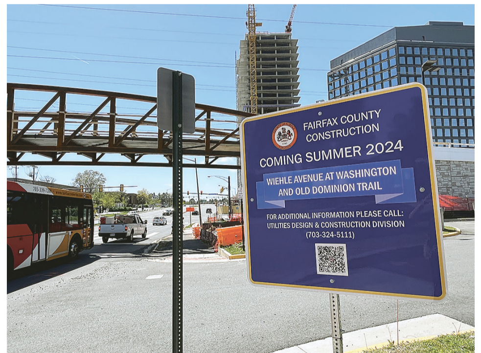
The bridge is not completed and operational yet.
