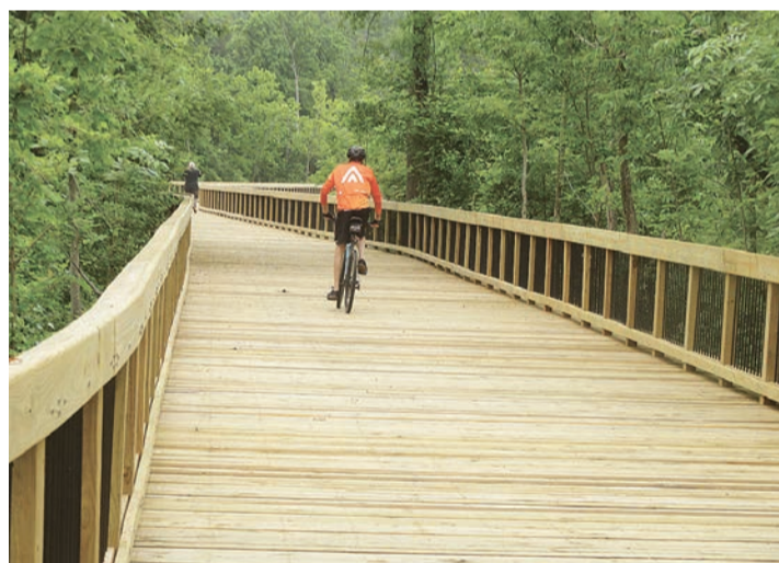
Bikers and walkers began to use newly-opened Bridge 23 immediately.
