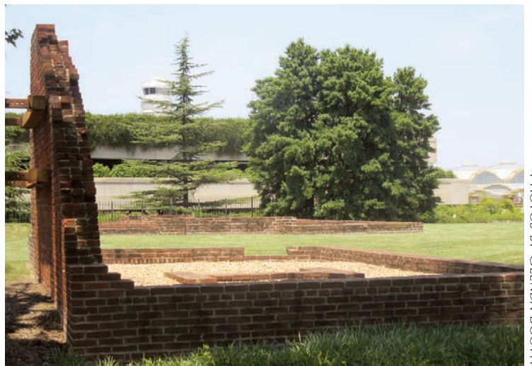
A juxtaposition, remains of the kitchen and laundry in the shadow of the airport’s control tower and terminals.
