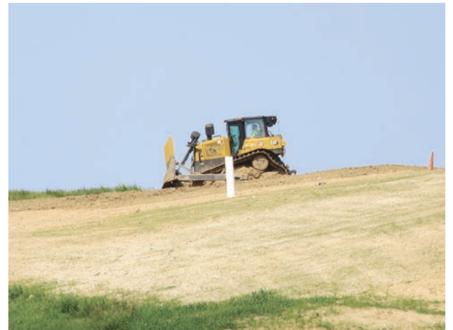
Big machinery rumbles around some sections of the landfill.
