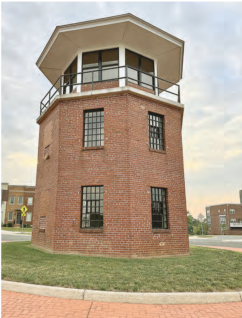
Guard towers dating from the Occoquan Prison years capture the style of a Medieval pavilion and now stand on repurposed prison grounds.
