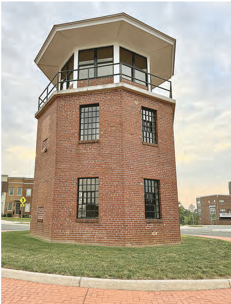
Guard towers dating from the Occoquan Prison years capture the style of a Medieval pavilion and now stand on repurposed prison grounds.
