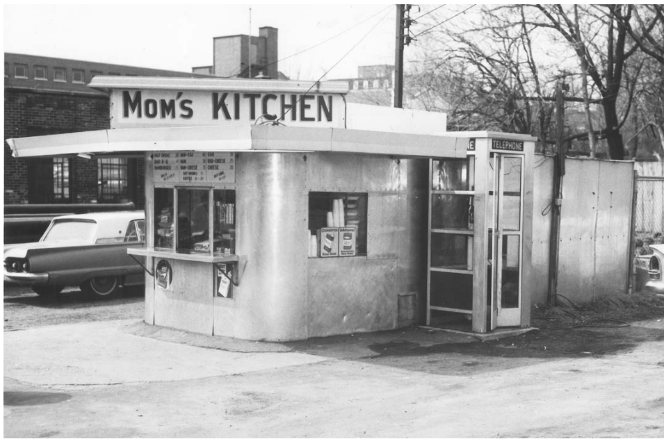
Williams restaurant, Mom's Kitchen, which stood on the corner Oronoco Street and Pitt Street
