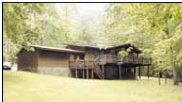
Clifton - $595,000 - Deck House w/ Pond
