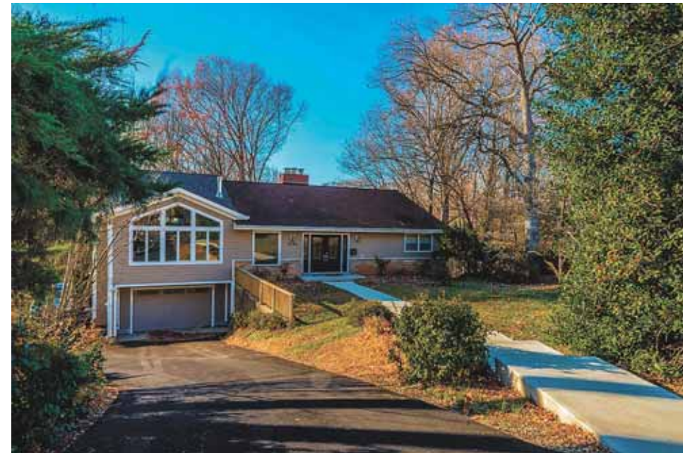
The 17.5-foot by 13-foot window wall that dominates the new side-facing gable is one component in a re-rationalized front elevation which now features a well-defined entranceway comprised of glass-facing French doors and sidelights.
